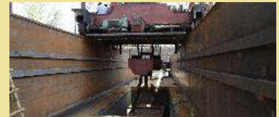
Load Testing Facility
