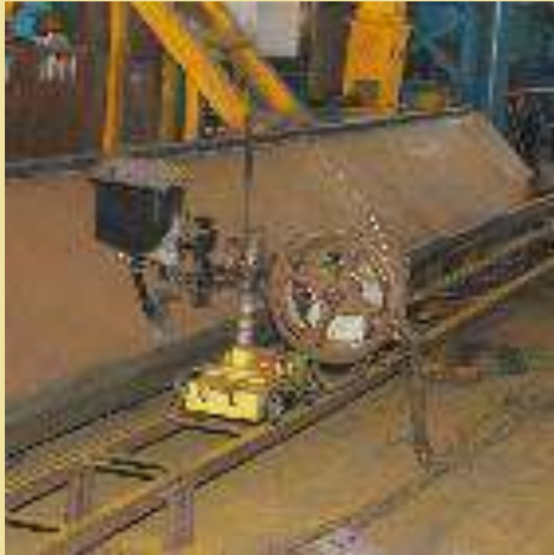
SAW Welding Shop
